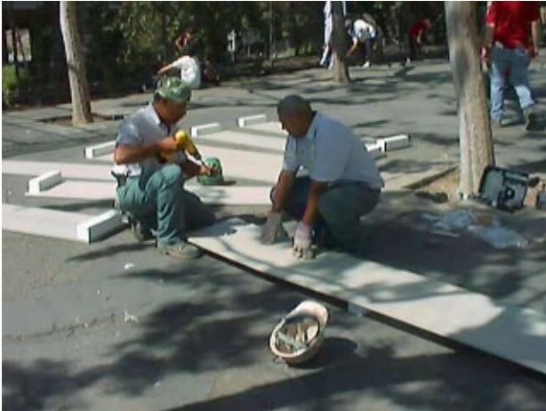
Raised beds being constructed of recycled plastic lumber.
