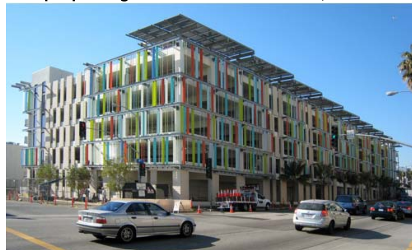
Sample parking structure in Santa Monica, CA
